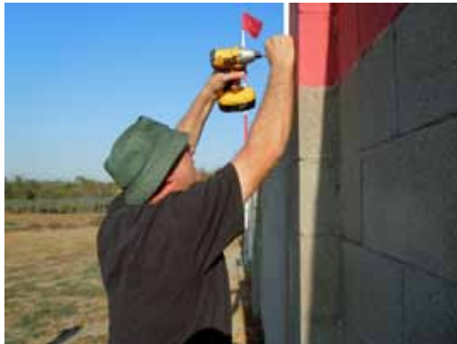
Jerry installing new flags on wall
